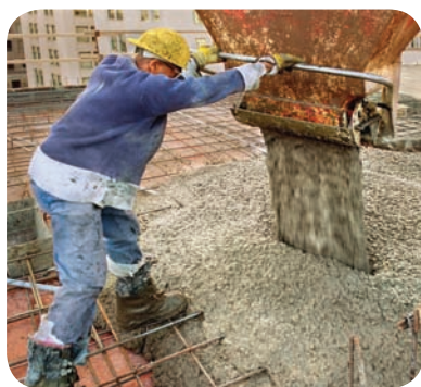
Figure 1 The steel rods (at the worker's feet) used to reinforce concrete are designed to expand and contract in the same way the concrete expands and contracts.
