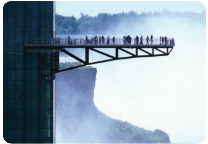
Figure 5 A cantilever is a beam that is supported at only one end.
